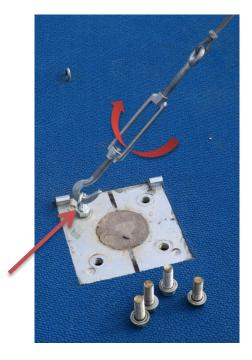
3. Before you proceed to the next step please make sure that the cage gate is properly fastened to the anchor with the hinge axis (item 7).
