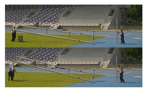
7. After the gate is lifted, fix the extreme pillar to the anchor.
