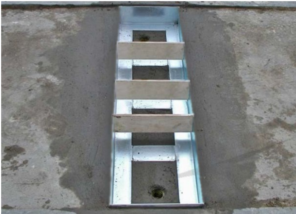
Image no. 1. Installed tray secured with spacing boards
