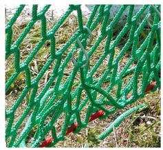
Next we put the net edge under the bottom net tension cable (item 6), strain the net and fix its edge to the meshes with supplied net hooks (item 7, drawing no. 5).
