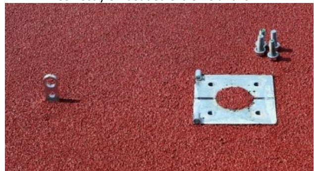
Correctly embedded extreme anchor
